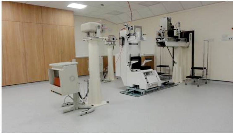
The treatment room at Clatterbridge
